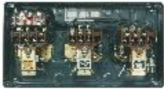
Interior View of MK2 FASD
