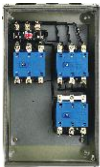
Interior View of ML SASD
