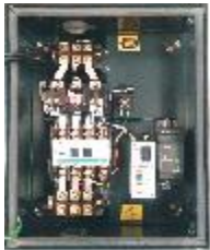
Interior View of MU-G10W DOL
