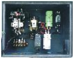
Interior View of MR-G2W
